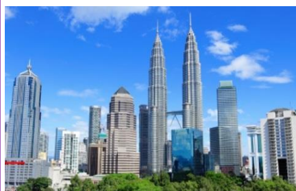
Pertonas Twin Tower
